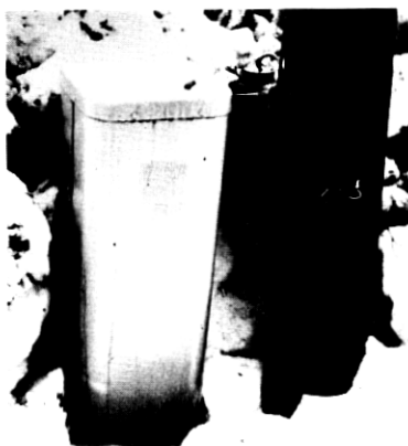
Fig. 19— SLC ™ -40 pedestal-mounted repeater enclosure.
