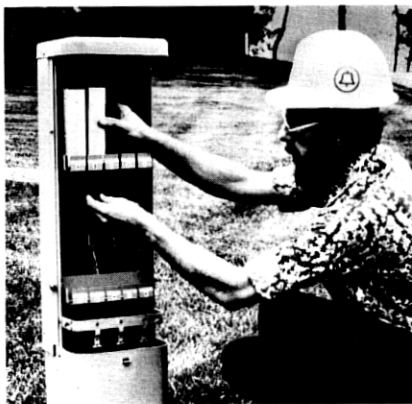
Fig. 19— SLC ™ -40 pedestal-mounted repeater enclosure.
